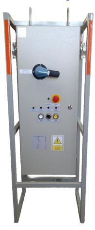
Switchgear type RKS4-1/4U is an electrical device designed for use in the underground mining pits in nonexplosive conditions and on the ground.
